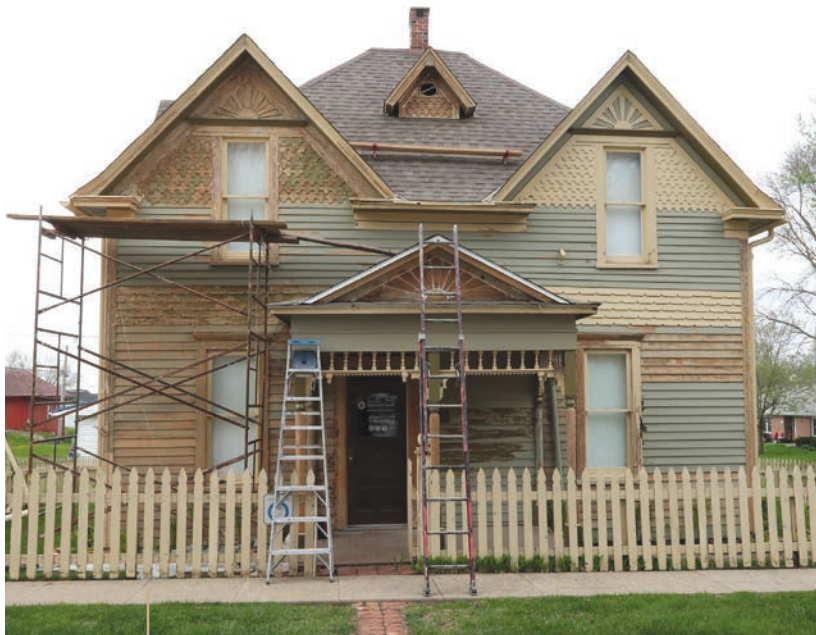
Figure 4 Front face of Bedstemor's House, north face with scaffolding in place and partial paint stripped
