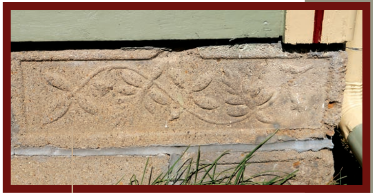
Figure 3 South face, cement foundation block with flower molding
