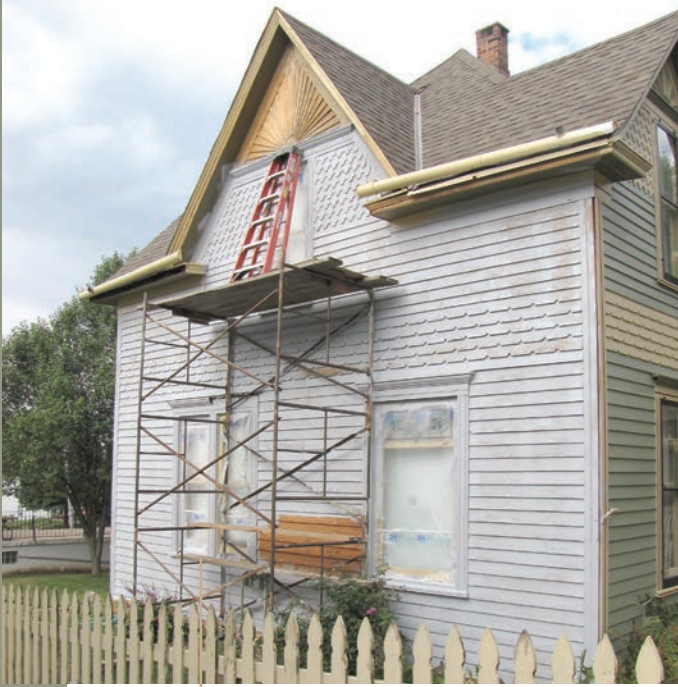
Figure 6 Bedstemor's House east face with primer coating
