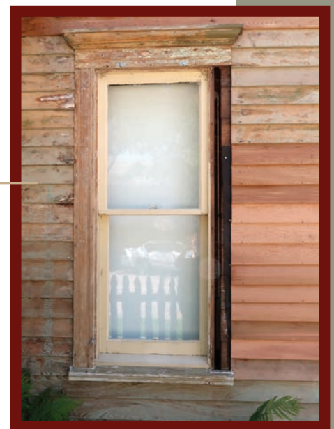
Figure 5 Bedstemor's House north face, wood siding, original and replacement pieces
