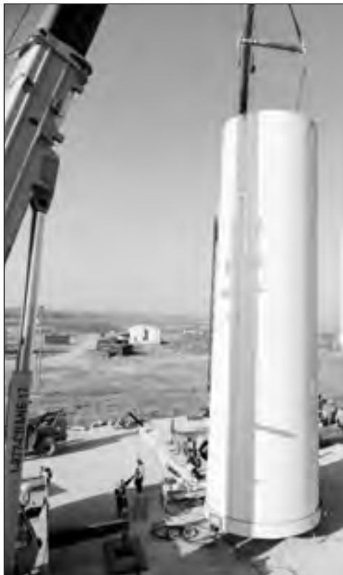
A wind turbine installation process.
